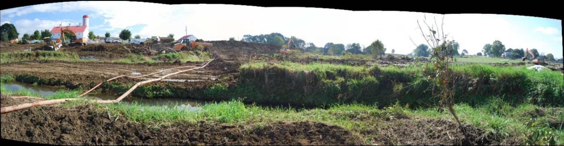
Restoration by LandStudies, Inc. , Lititz, PA
